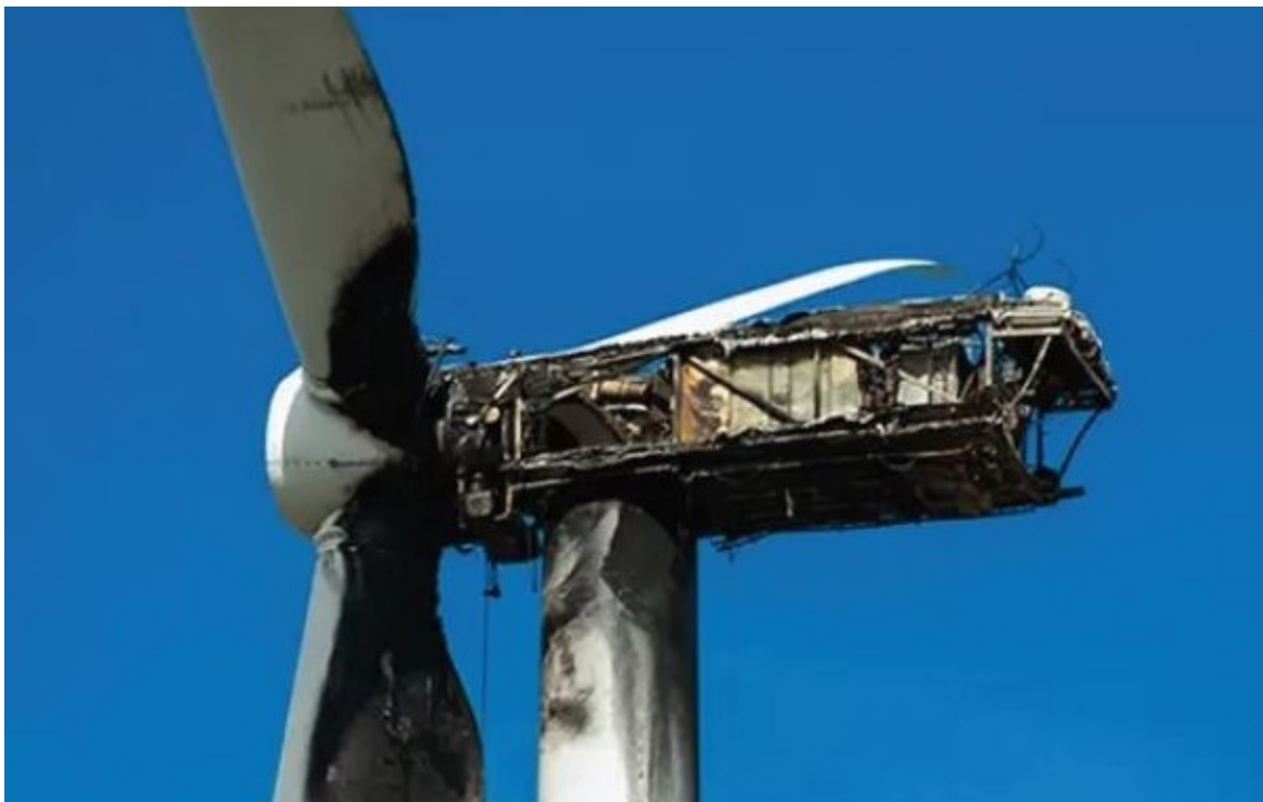
Figure 12 Wind Turbine With Damaged Nacelle Showing Extensive Oil Leakage ( LAIER -Oil Leaks in Wind Turbines: The Dirty Side of Clean Energy )
